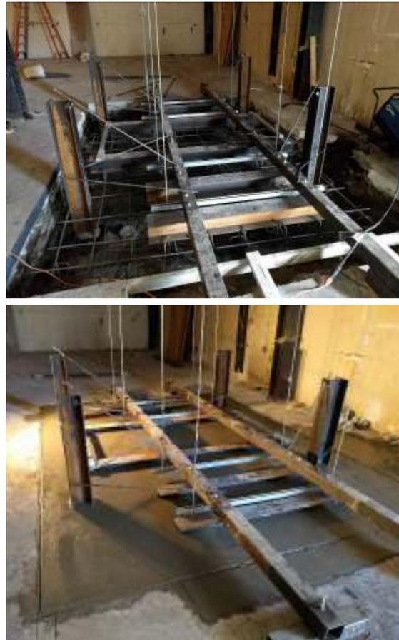
*Figure 13. Concrete base. Top: sub-frame structure. Bottom: Concrete poured*
